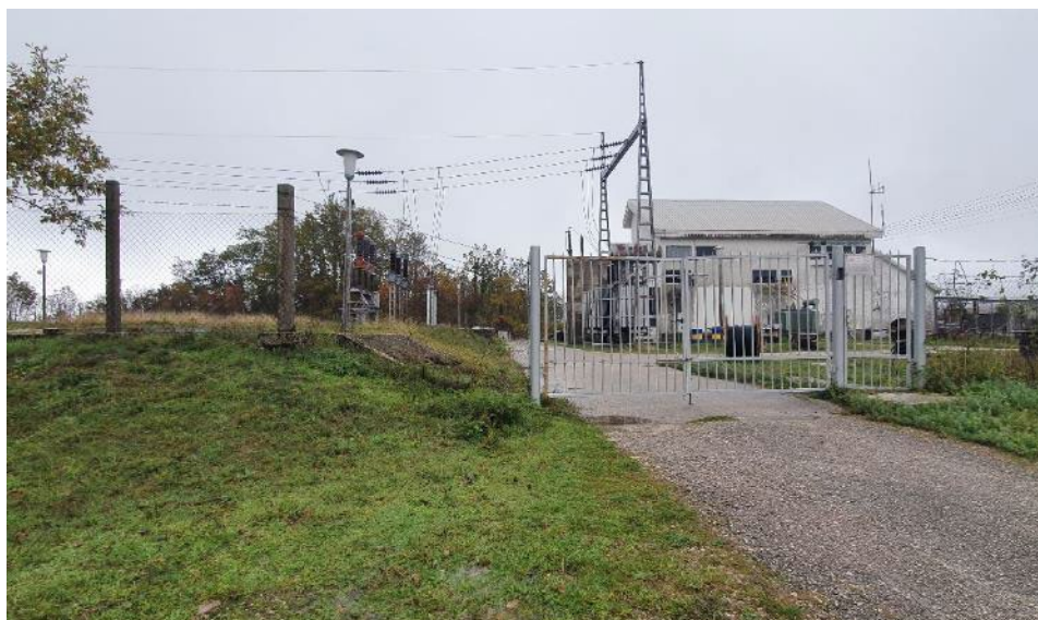
Figure 8-4: Photograph of SS Vilusi entrance (Source: Enova)
